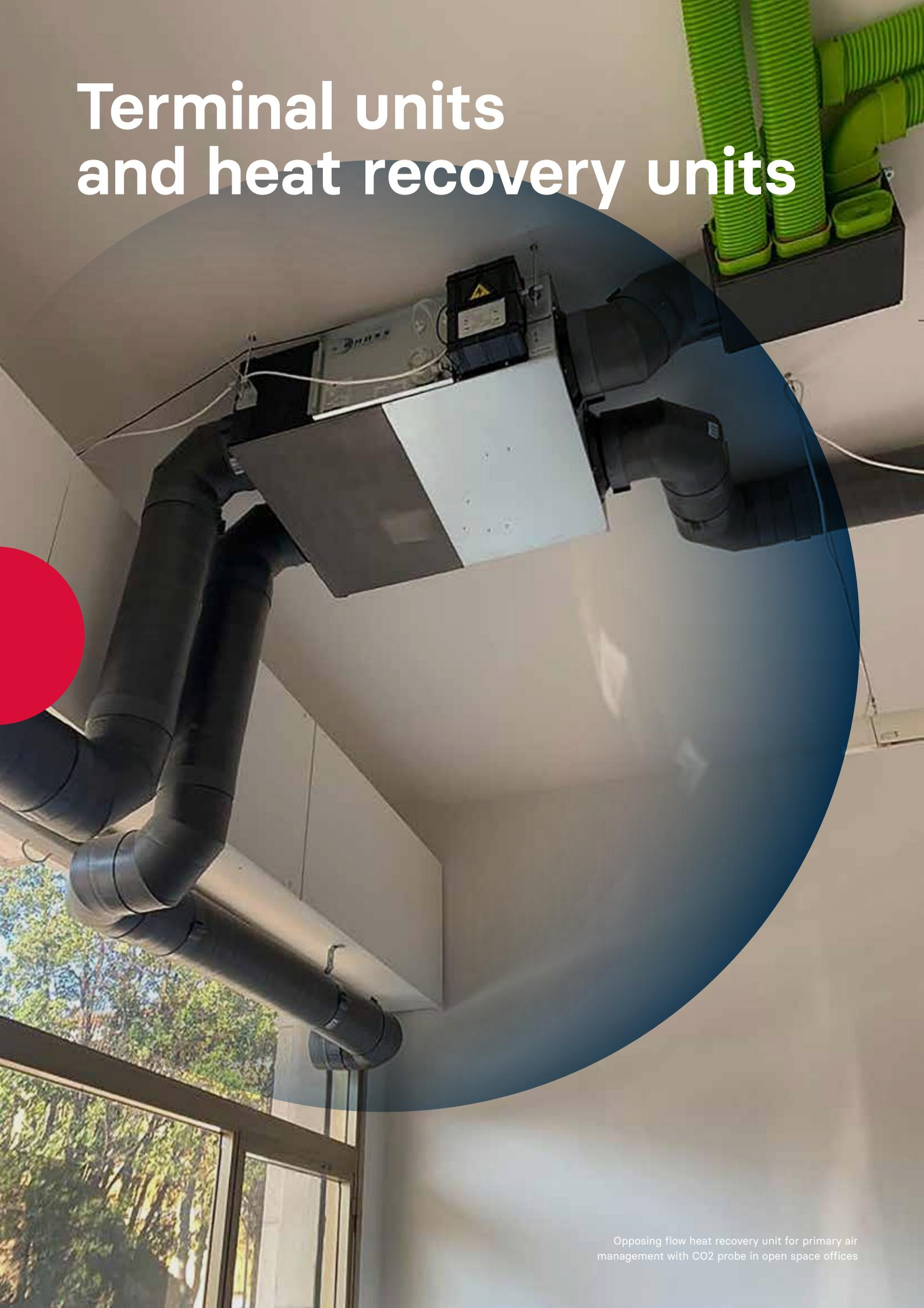
Opposing flow heat recovery unit for primary air management with CO<sub>2</sub> probe in open space offices
